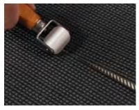
8. Refold the strips, carefully joining the two edges for a smooth seam and ensure the seal with the seam roller; then smooth out the entire area with the heavy roller to remove any air bubbles.
