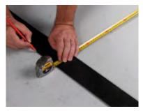
**3.** Mark the exact position of the initial strip while making sure to leave enough room in both directions for the levelling.
