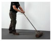
**10.** Press firmly into place, working out any air bubbles with the smoothing roller. Fold up the other side of the strip and repeat steps 6, 7, 8 and 9.
