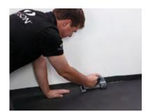
**9.** Cut the outer edges of the floor covering to fit the shape of the room, following along the walls, baseboards, pipes and other notches as closely as possible:
