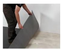
**7.** Observe the appropriate flash time, then lay the flooring strip into the adhesive.
